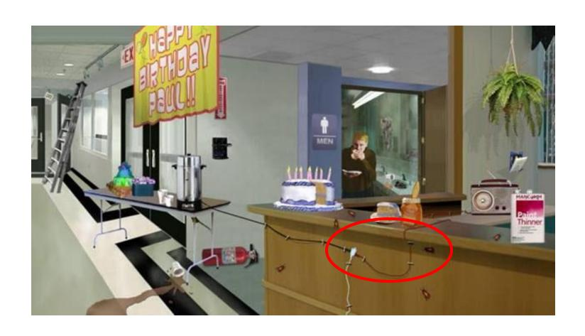
Radio extension cord is stapled to the counter. Flexible cords may not be used where attached to building surfaces.
